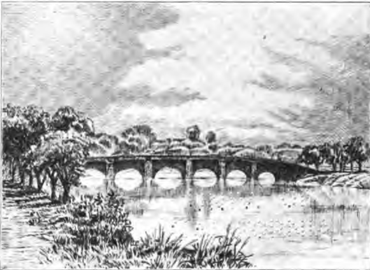
BRIDGE OVER THE COOUM NEAR GOVERNMENT HOUSE.
