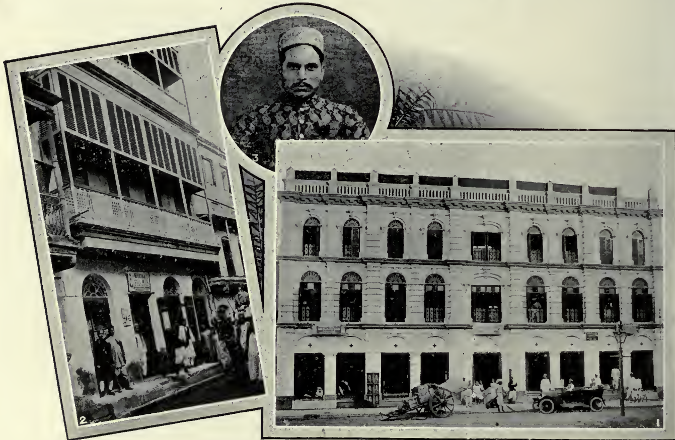
1. EXTERIOR OF NEW PREMISES,
