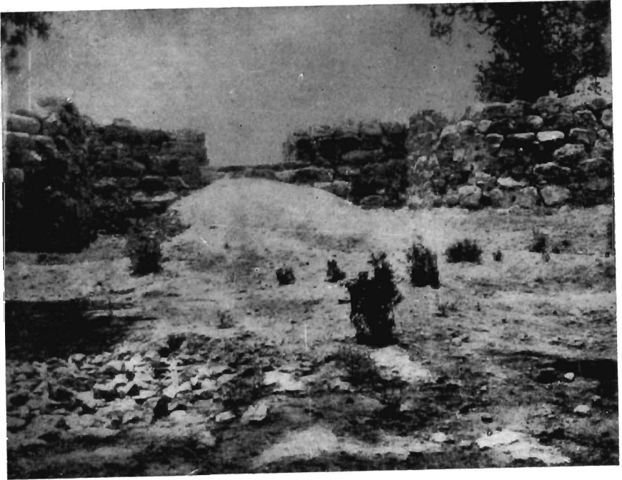
Fig. 2. Rājagriha: Rampart walls of cyclopean masonry.
