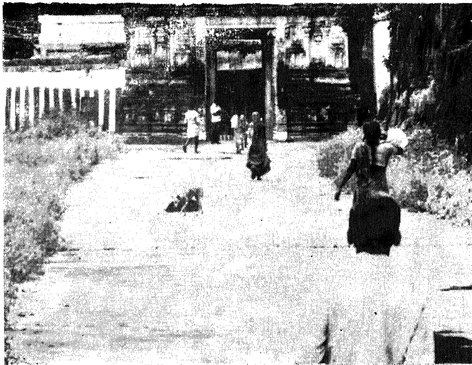
PLATE 29 : Rajagopuram ( before renovation )
