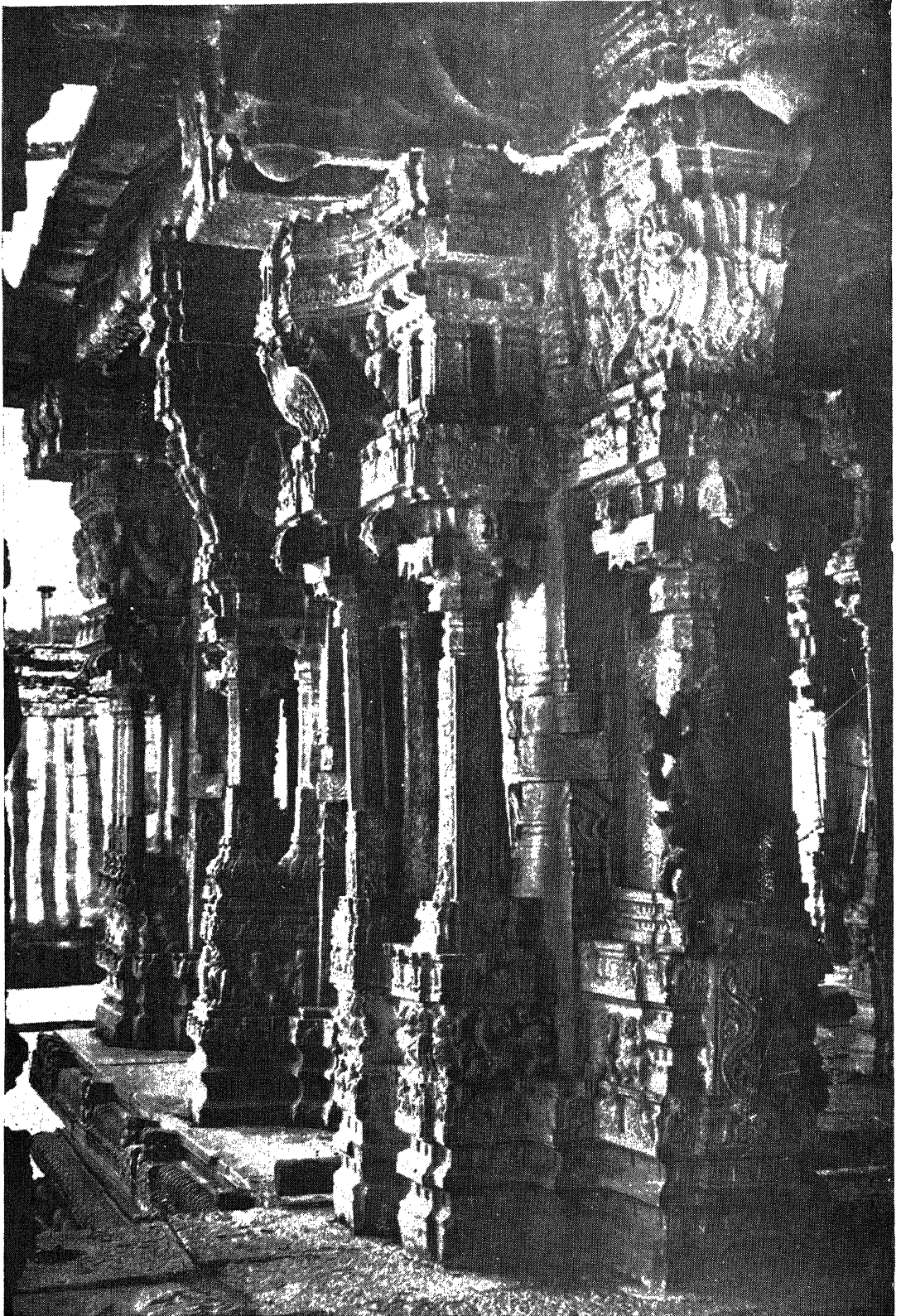
PLATE 65 : Vijayanagar pillars with corbels and well developed 'Pushpa bodigais'
