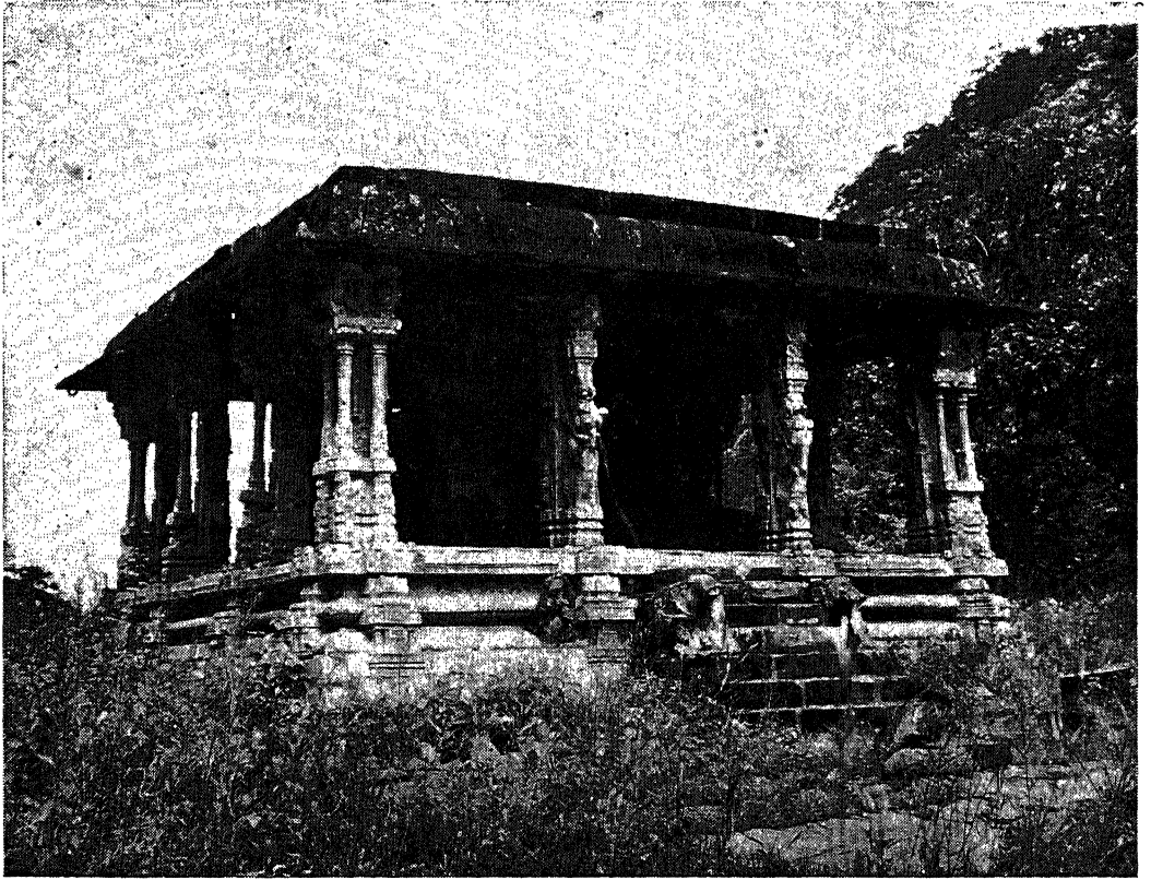
PLATE 23 : Udyogamantapam on Upper Ahobilam ( Before renovation )
