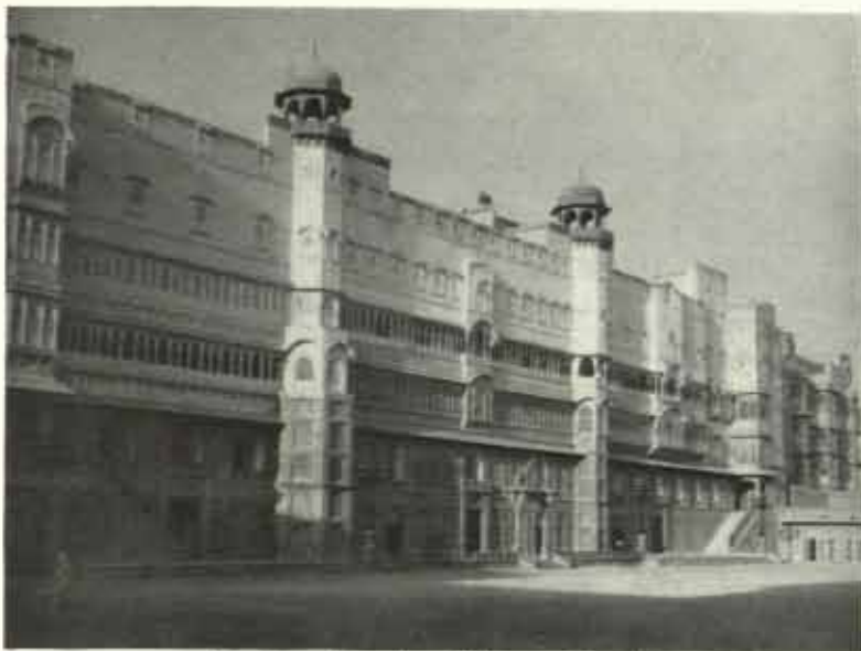
31. Northern Façade of Bikānēr Fort Palace.
